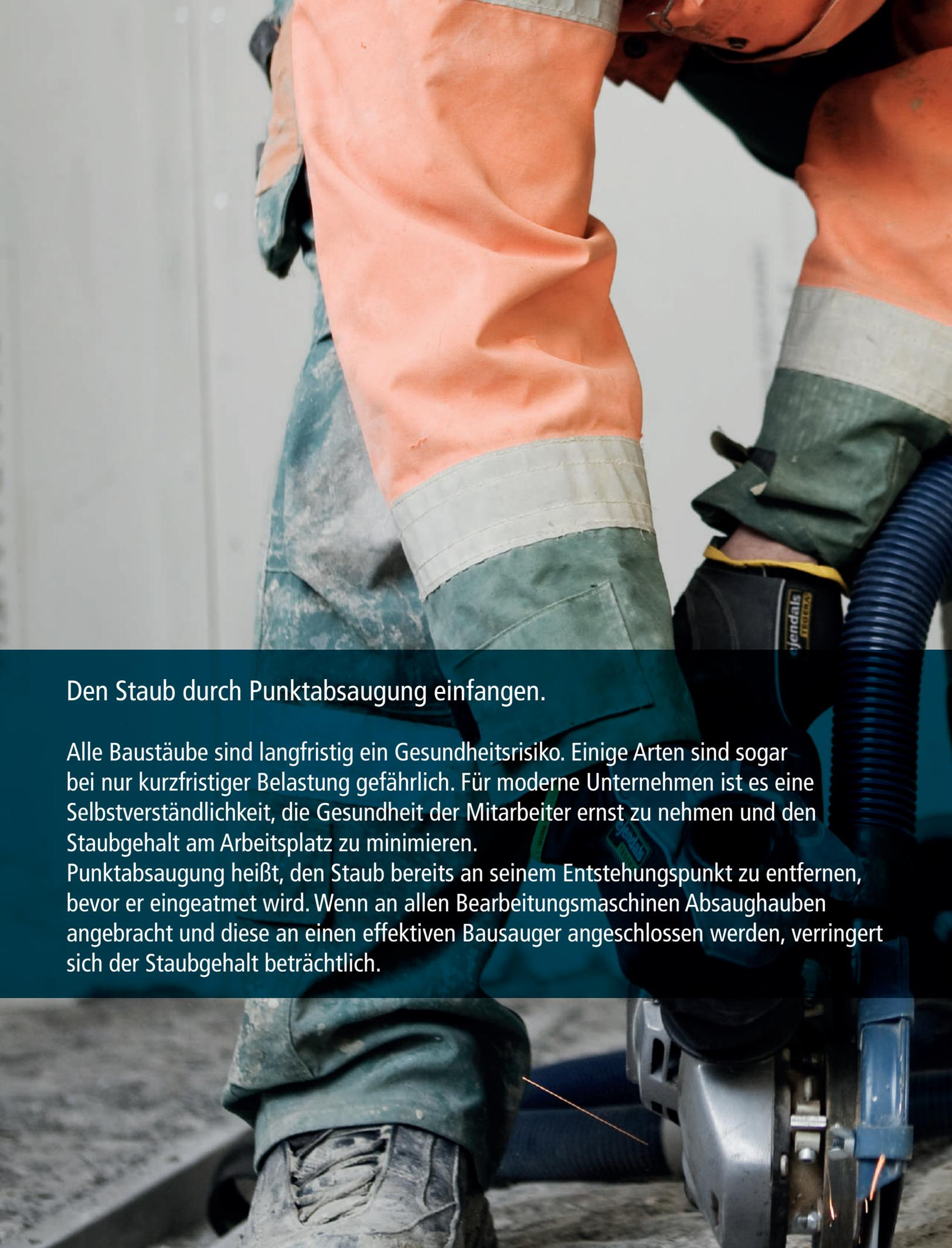
A close-up photograph of a worker wearing orange safety overalls and green protective sleeves. The worker is using a blue power tool, likely a circular saw, which is equipped with a dust extraction system. A blue corrugated hose is connected to the tool, and a thin orange laser line is visible on the ground. The background is a plain, light-colored wall.
