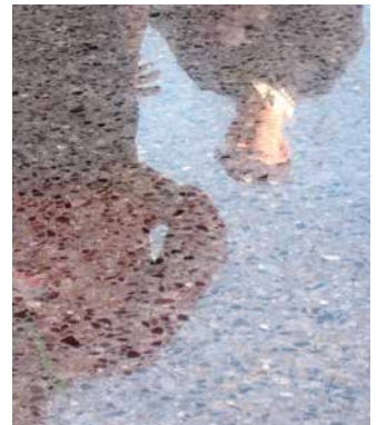
Beton polieren (Crystal finish)
