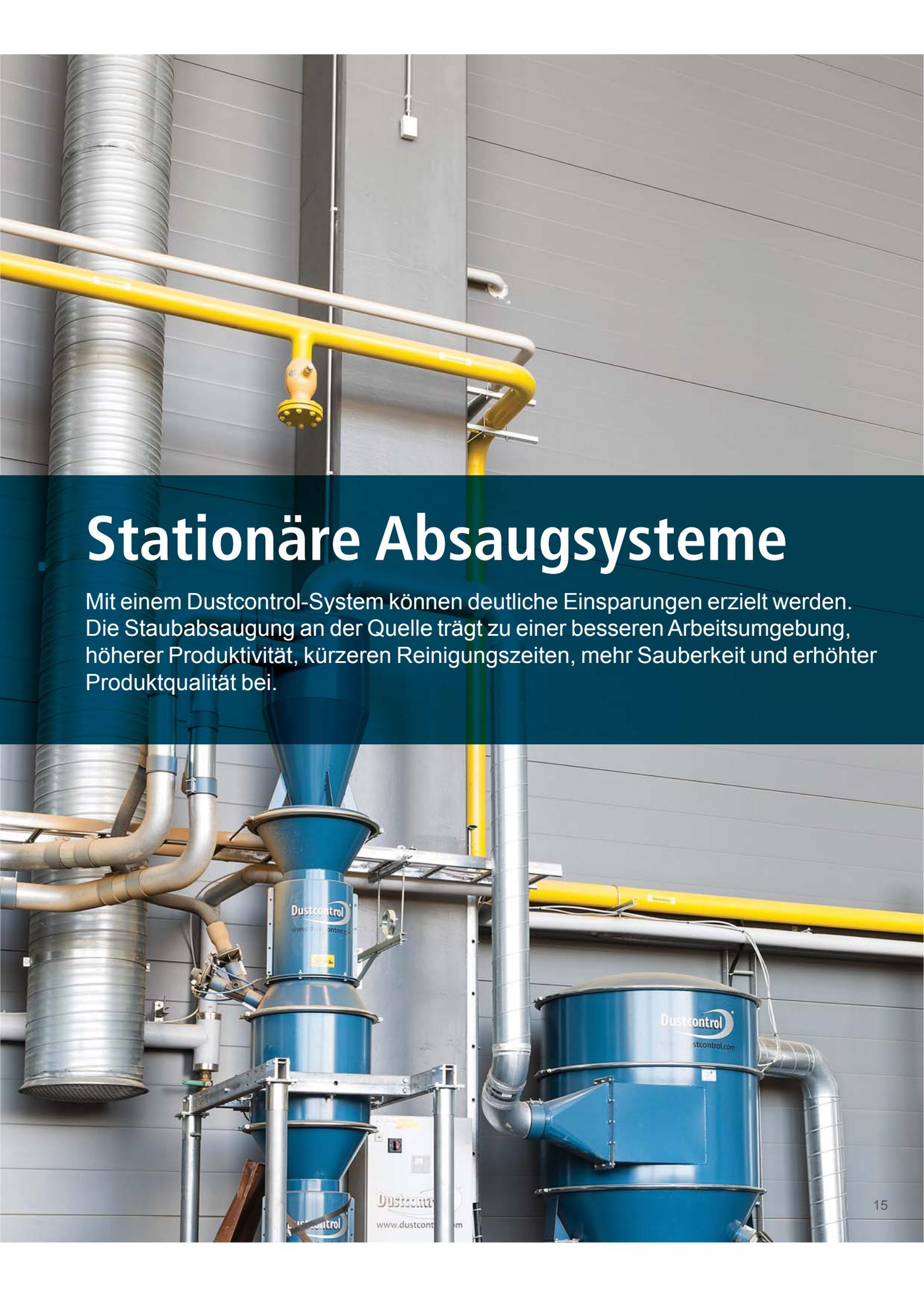
The image shows a complex industrial dust extraction system. A large, vertical, corrugated metal duct is on the left. A network of yellow pipes runs horizontally across the upper part of the frame. Below this, a blue Dustcontrol cyclone separator is mounted on a metal frame. To its right is a larger blue Dustcontrol bag filter housing. The background is a grey industrial wall with various pipes and electrical conduits.
